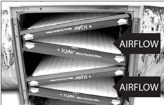
7. Double check that all filters have been inserted correctly and replace access panel with screws.
