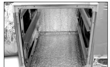
6. Remove filters and secure via panel from inside to the air handler.
