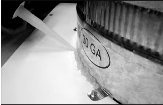
9. Seal the gap between the collar and the panel and wait till it is dried.
