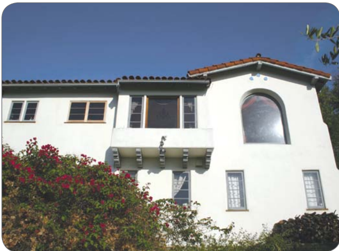
10 This home's air quality was improved by over 95% within 90 minutes of installation, and that's a typical result.
